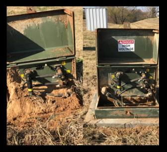
URS will be cleaning and clearing inside and around the underground equipment. This will help maintain the reliability, lifespan and safety of our equipment. Above is an example of work they have done in the past at other electrical companies. These are not pictures of SBEC equipment.
